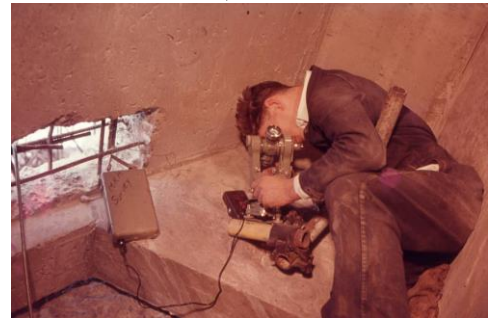
Figure 1 Sydney Opera House original model and drawings showing element information. Bottom right: Stations inside the arch were used when jacking the side shell arches to correct errors due to the compression of the formwork. The instrument is bolted to the shear pin linking the segment to the concrete below (Elfick, 2010).
